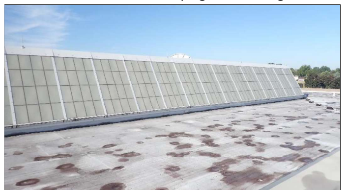
Overview of skylight structure
