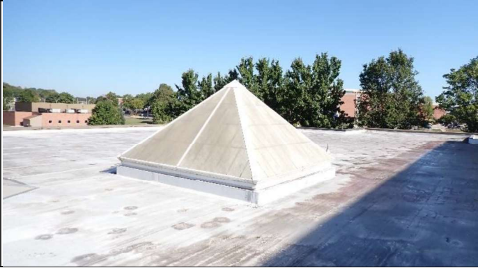
Overview of skylight structure
