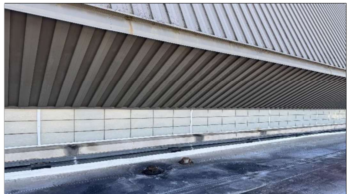
Overview of limestone coping above dining area
