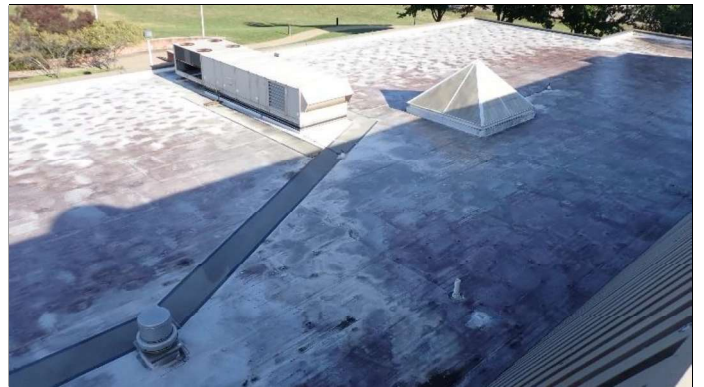
Overview of low-slope roof
