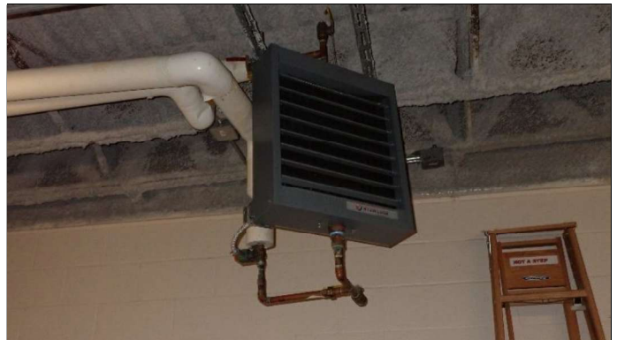
Convection unit heater
