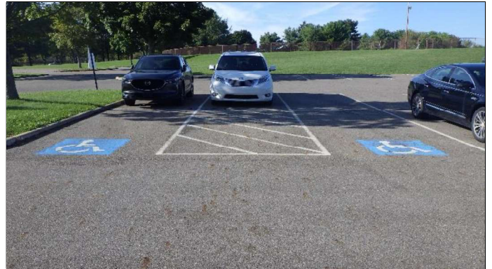
Overview of accessible parking with no signage
