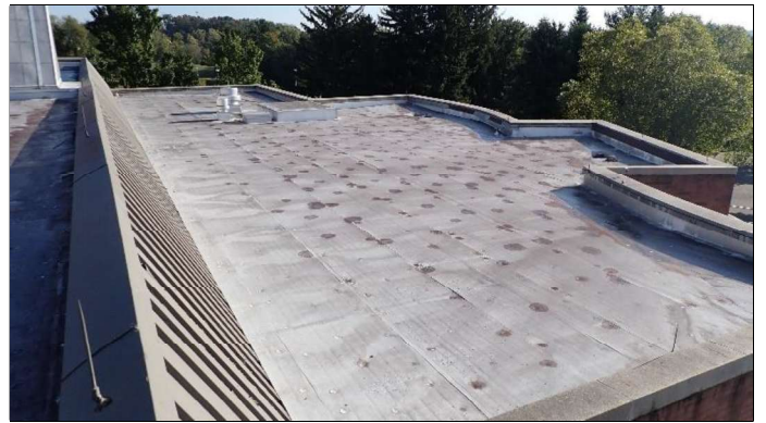
Overview of low-slope roof
