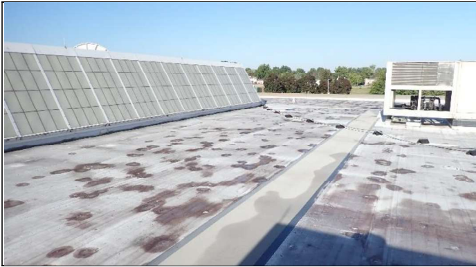
Overview of low-slope roof
