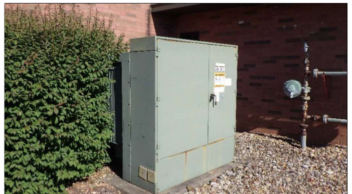
Pad-mounted transformer
