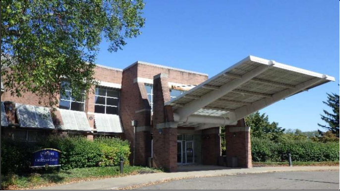
Overview of typical porte-cochere
