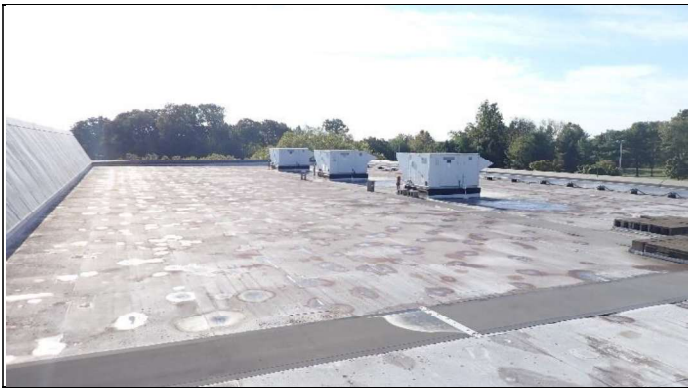
Overview of low-slope roof
