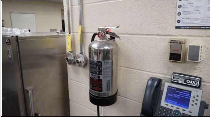
Wet chemical fire extinguisher
