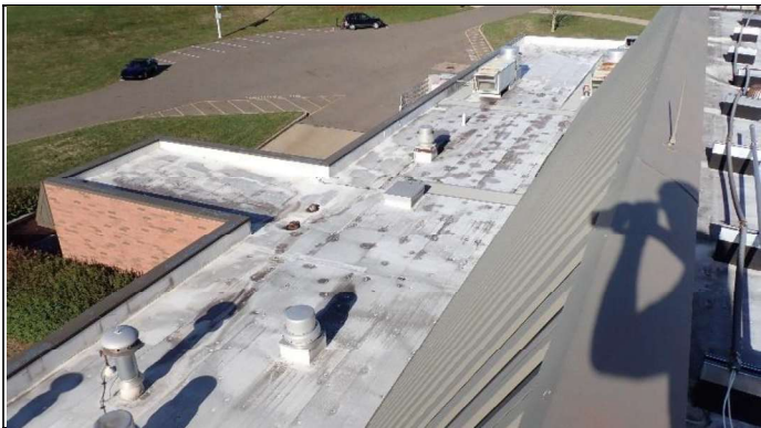
Overview of low-slope roof
