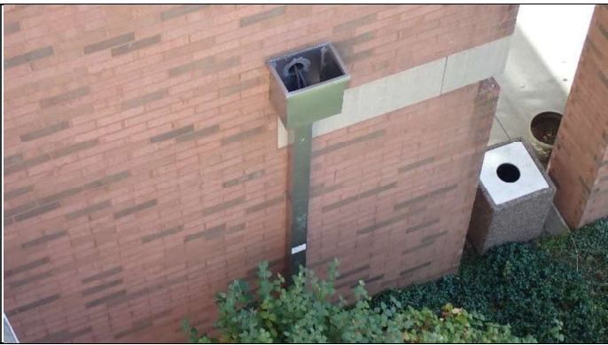
Scupper and downspout
