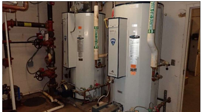
Tank-style water heaters
