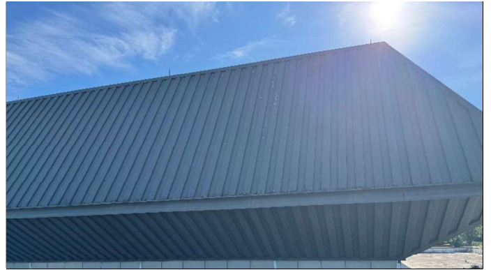
Overview of mansard roof
