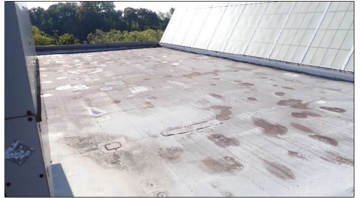
Overview of low-slope roof
