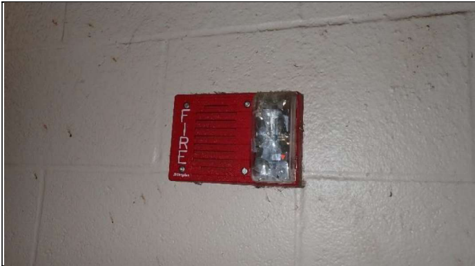
Typical strobe/siren fixture
