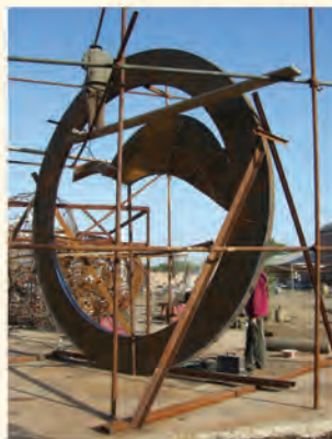
Construction of "Rings of Unity — Circles of Inclusion" at the Beijing site.
