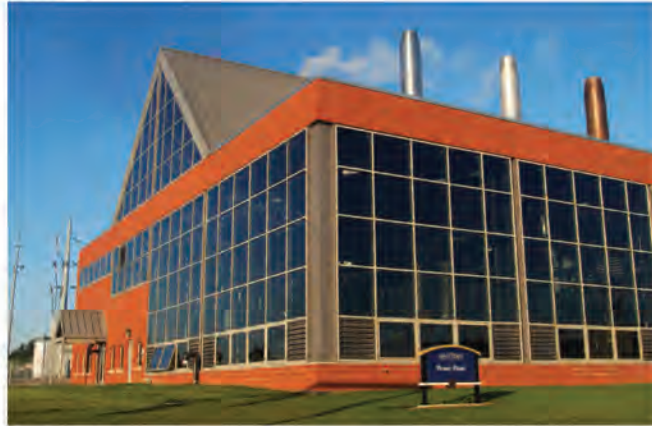
Located on Summit Street, Kent State's Power Plant supplies steam, electricity and air conditioning to Kent Campus buildings.
